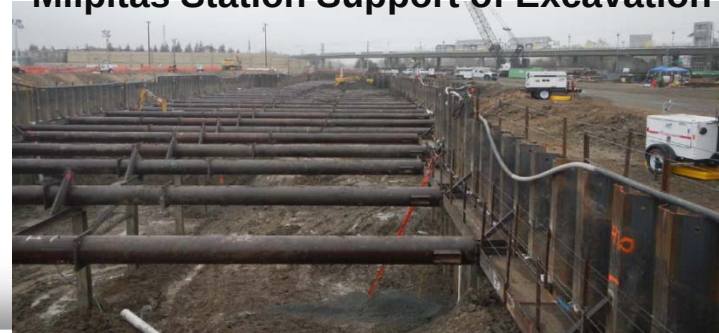
Milpitas Station Support of Excavation
