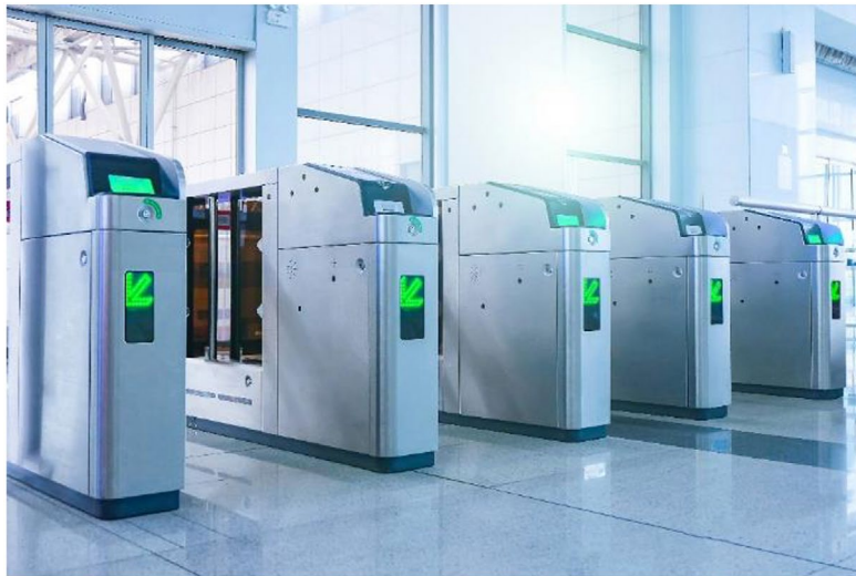
Figure 3-12 Customer-Facing Fare Collection Assets at a Transportation Hub
